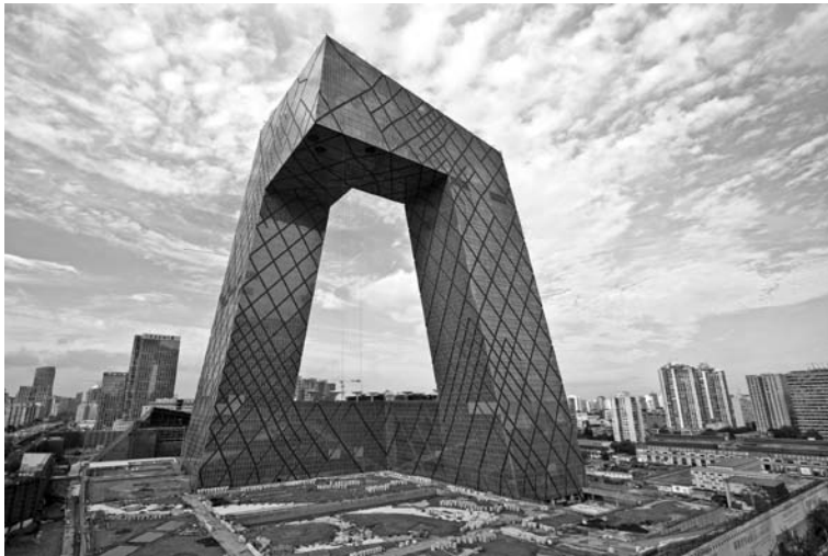
FIGURE 1.11 CCTV Tower. (Photo by ARUP.)
