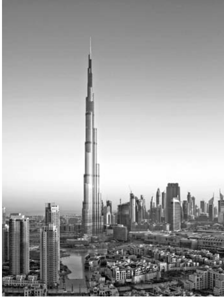
FIGURE 1.12 Burj Khalifa. (Photo by SOM/Nick Merrick © Hedrich Blessing.)
