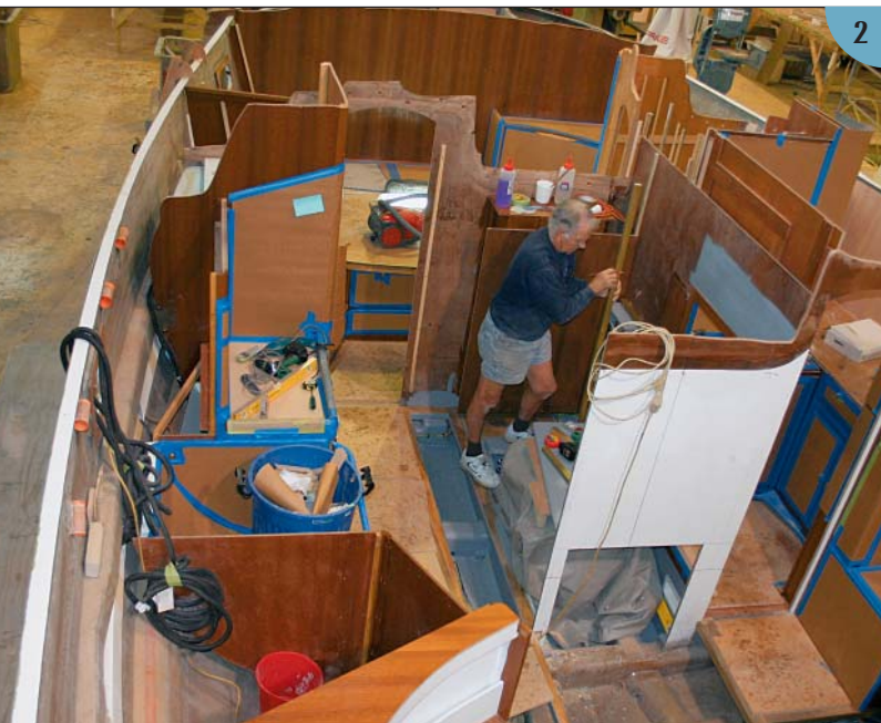
(2) On larger boats the interior may be made in a furniture shop and fitted to the boat while the deck is still being made. Here the components of the cabin spaces can be easily seen.
