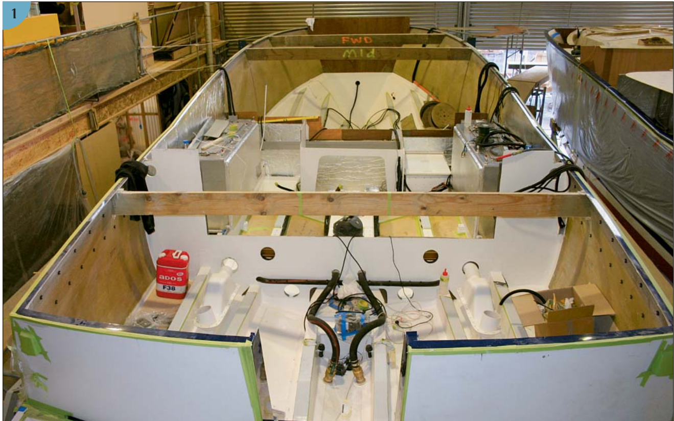
(1) The interior of this boat is being fitted out before installing the deck. This procedure cuts down on the time needed
