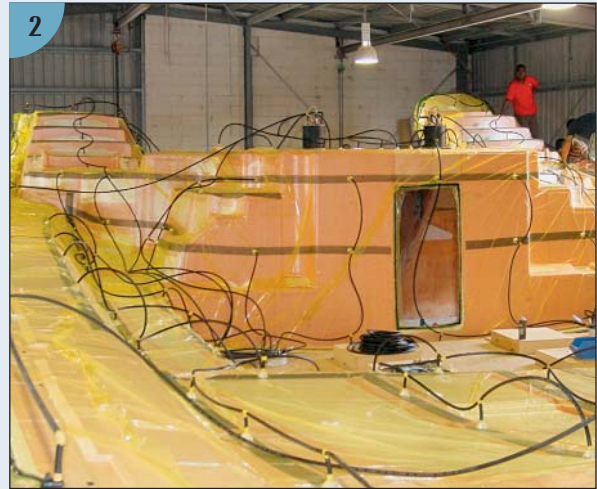
The infusion lines are in place, and as soon as the vacuuming is completed, the valves will be opened and resin will pass through the larger-diameter lines into the laminate. (Courtesy Perry Catamarans, Queensland Composites, and High Modulus)
